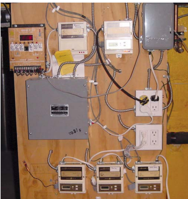
The central mounting board for various GL-30s and the old GL-100 used for monitoring, along with a box containing relays for geothermal control.
