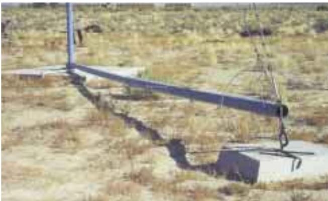
required for various tower heights and soil conditions. Why is this important? Putting the concrete in and getting the schedule 40 pipe cost nearly the same as the wind generator.
